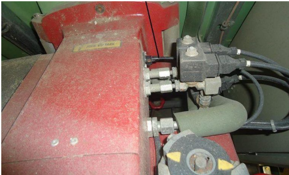
Picture 2 – Incinerator construction
