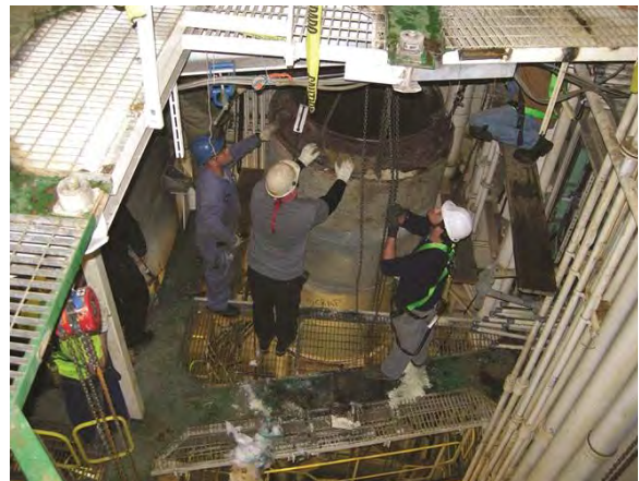
Figure 3. Removal of the existing exhaust gas silencer sections.
