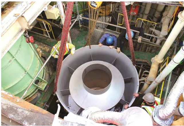
Figure 2. Rigging the scrubber section into the ship.
