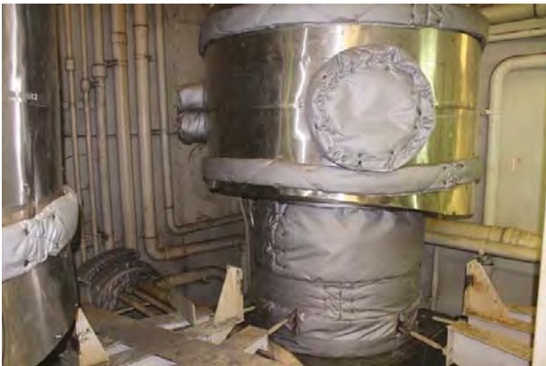
Figure 5. The fully insulated and cladded scrubber section in position on board ship.
