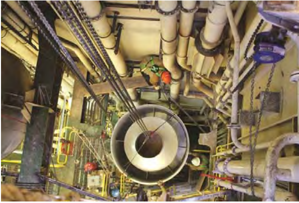
Figure 4. Lowering the scrubber section into place.
